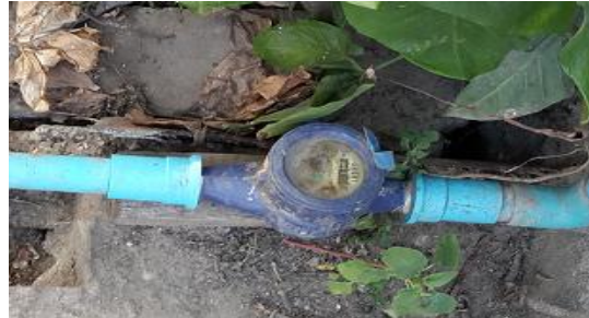
OLD WATER METER
